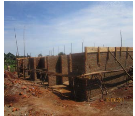
Above, ongoing construction at Budondo medical centre
