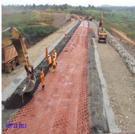
Right Embankment nearing Completion
