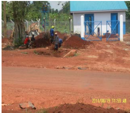
Construction of the waterline booster pump house in Naminya
