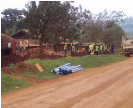
Laying of pipes for the water line project in Budondo
