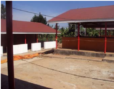
The newly constructed market in Malindi
