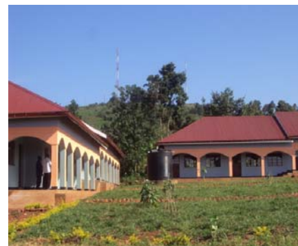
The ten classroom block constructed at Naminya RC Primary School
