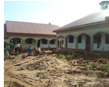
10 classroom block being constructed at Naminya RC primary school
