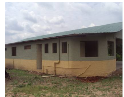
Completed and painted rafting takeout structure for NRE
