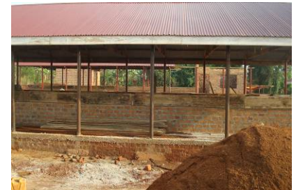
The market under construction
