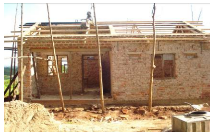
The Budondo Business Centre premises under renovation
