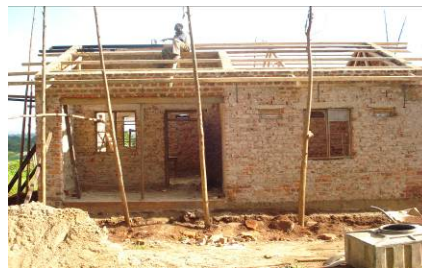
The Budondo Business Centre premises under renovation
