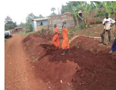
Laying of pipes for the water line project in Budondo
