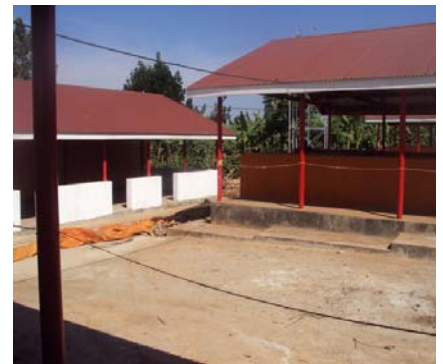
The newly constructed market in Malindi
