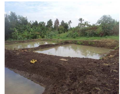
Above, the three community fish ponds excavated at Naminya
